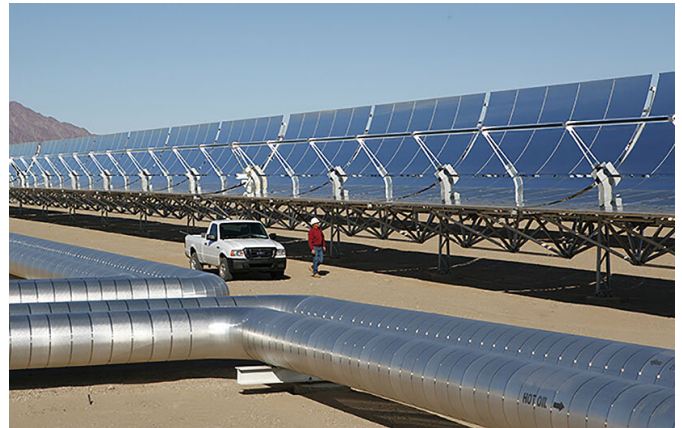
A partial view of the nearly 20,000 receivers at the Nevada Solar One power plant in Boulder City, Nevada. Credit: Nevada Solar One
