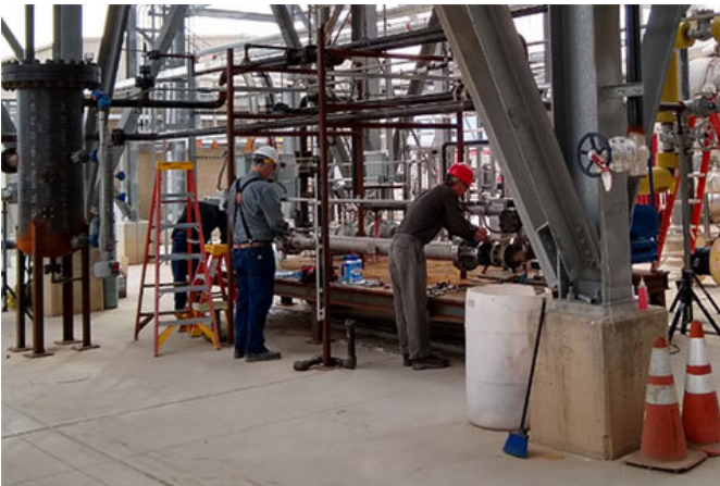
Installation of the integrated hydrogen sensor/separator module at Nevada Solar One. Credit: Koenraad Beckers, NREL
