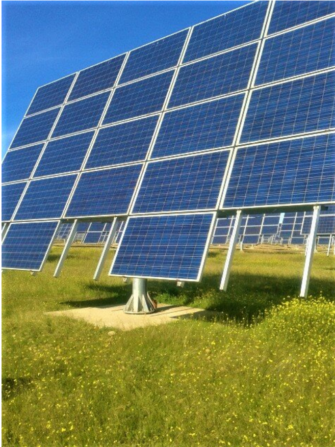
Solar tracking designed by the University of Cordoba. Credit: Universidad de Córdoba
