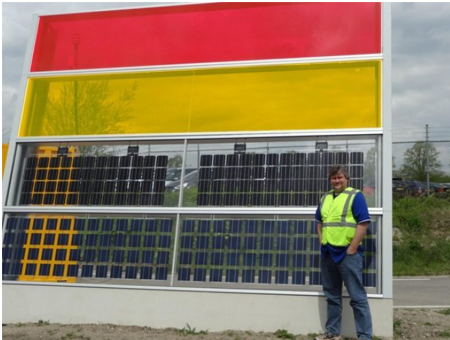
Michael Debije standing next to part of the Solar Noise Barrier project, which stood in Den Bosch 2015-6. Credit: Eindhoven University of Technology
