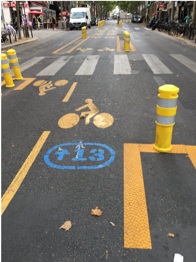
The 'Velopolitain M' pop-up cycling lane on the Avenue de Saint Ouen in Paris. It designed to follow the city's number 13 metro line, allowing former or occasional subway users to easily find their way when cycling. Credit: Chris93/Wikimedia , CC BY
