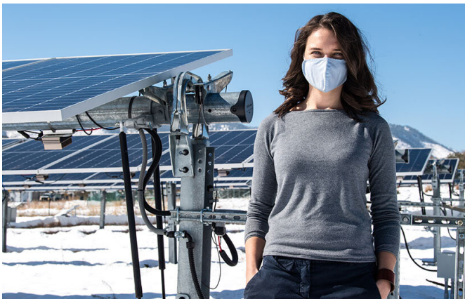
NREL researcher Sarah Toth stands next to a PV tracking system at NREL. Like any PV system, these attract dust. Toth has developed sensors to measure real-time soiling ratio and installed some in Los Angeles. Credit: Dennis Schroeder, NREL
