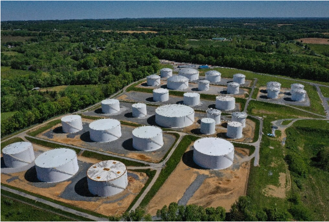
Fuel holding tanks are seen at Colonial Pipeline's Dorsey Junction Station in Woodbine, Maryland on May 13, 2021.
