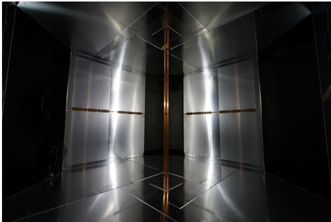
The wireless charging room under construction at The University of Tokyo. Credit: The University of Tokyo
