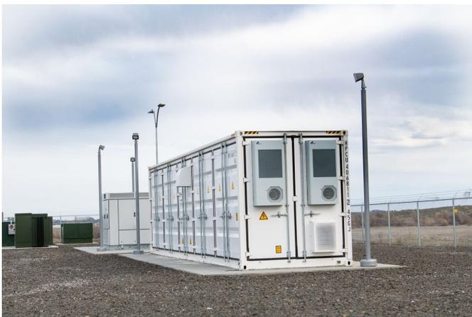
Battery storage at Pacific Northwest National Laboratory's solar array. Batteries are a critical component of microgrids, which also often include backup generators to withstand emergency outages during a broad range of weather conditions. Credit: Andrea Starr | Pacific Northwest National Laboratory
