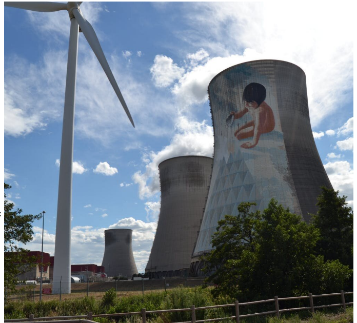
Cruas nuclear power station in southern France. Credit: Jean-Pierre Pertin
