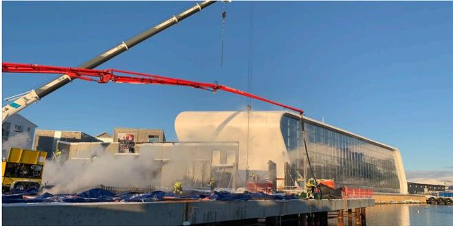
Winter casting using VIP elements in the quay at Hotel Richard With in Stokmarknes. Using the newly-developed system, a single machine can heat twice the area possible with surface-mounted pipes. Credit: Tommy Holan/Betong & Entreprenør
