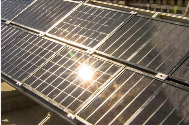
The graphene-perovskite solar panels installed in Crete. Credit: Pescetelli et al.
