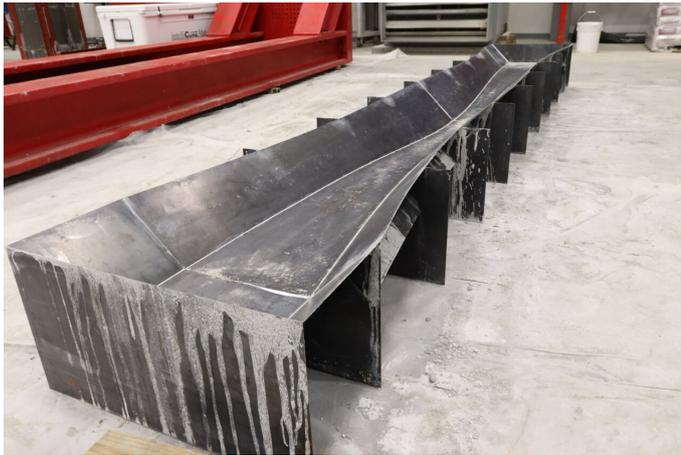
Formwork designed through the Zip-Form system allowed a concrete beam to be poured using less concrete but maintaining strength. Credit: Cameron Murray
