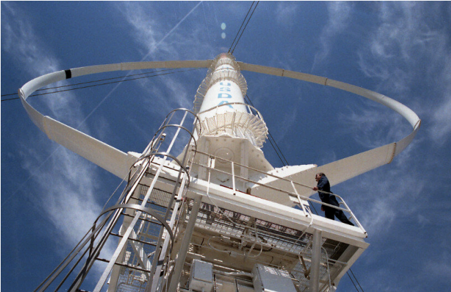
A historical photo of Sandia National Laboratories' experimental 34-meter-diameter, vertical-axis wind turbine built in Texas in the 1980s. Credit: Sandia National Laboratories
